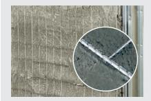
Cement plastering does not fall because it is hold by the knurled thick mesh\* (25 x 50 mm) placed in between the plate and the edge of the cement plastering.
